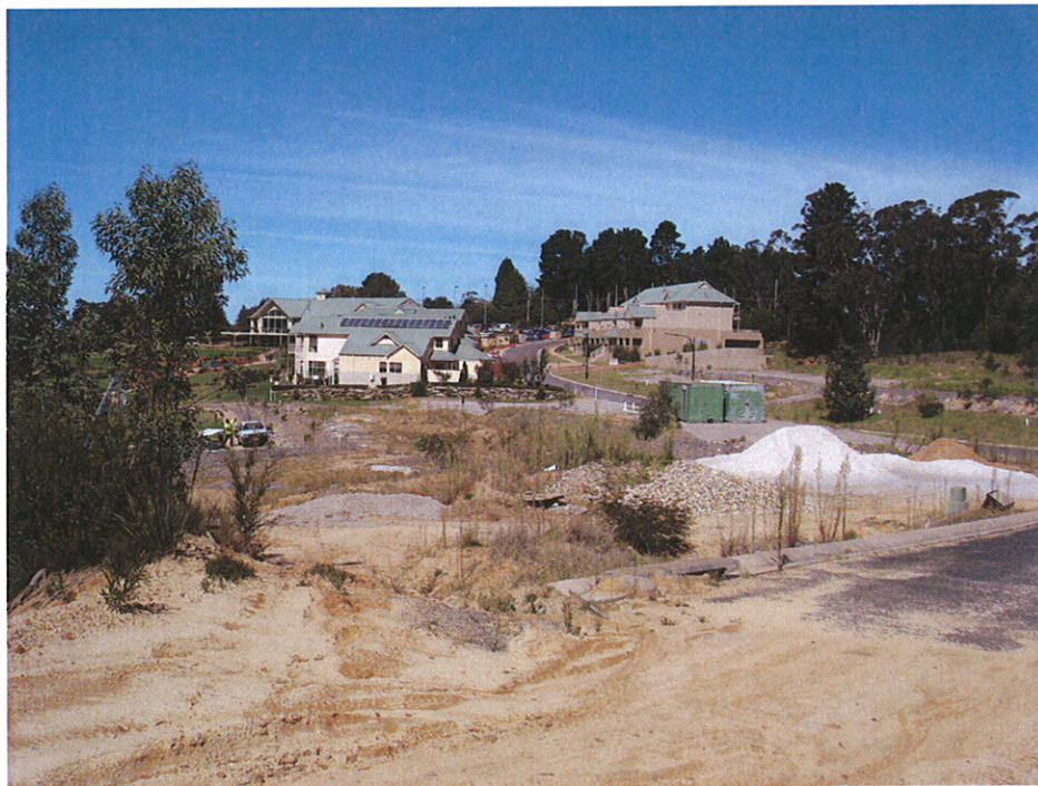
Existing Stage 1 residential development with earthworks for Stage 2 in foreground
